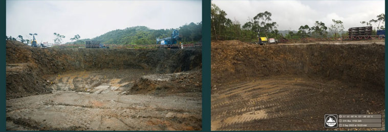
PLATFORM CONSTRUCTION (WTG20)
