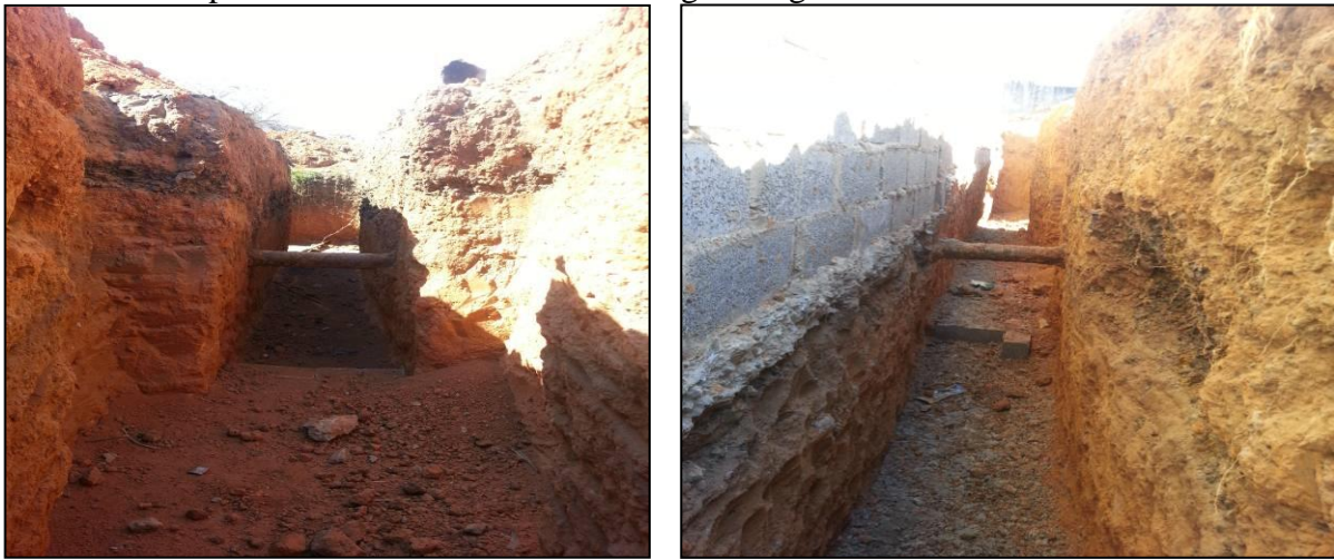
Photo 5: Example of Land Allocation on existing underground Services
