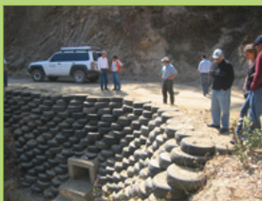
... terraces and protective walls made from old tyres to protect farmland and roads
