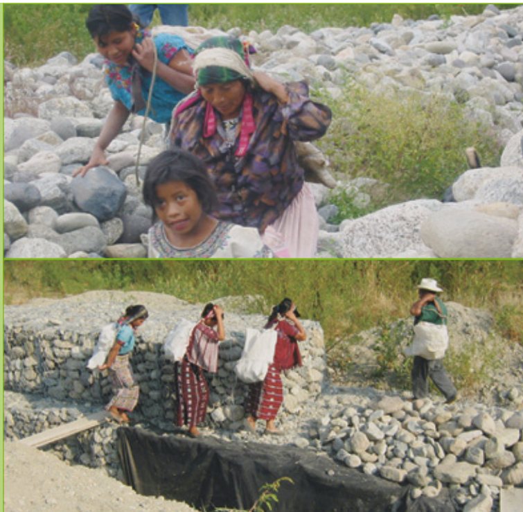
Bank reinforcement to protect settlements, agricultural and forestry areas from floods
